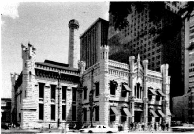
Like the Water Tower, the Chicago Avenue Pumping Station is castellated Gothic in style. (Bob Thall, photographer)
